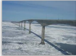
Confederation bridge Canada - 1997
