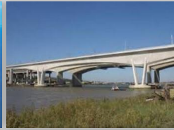
Medway bridge UK - 2001
